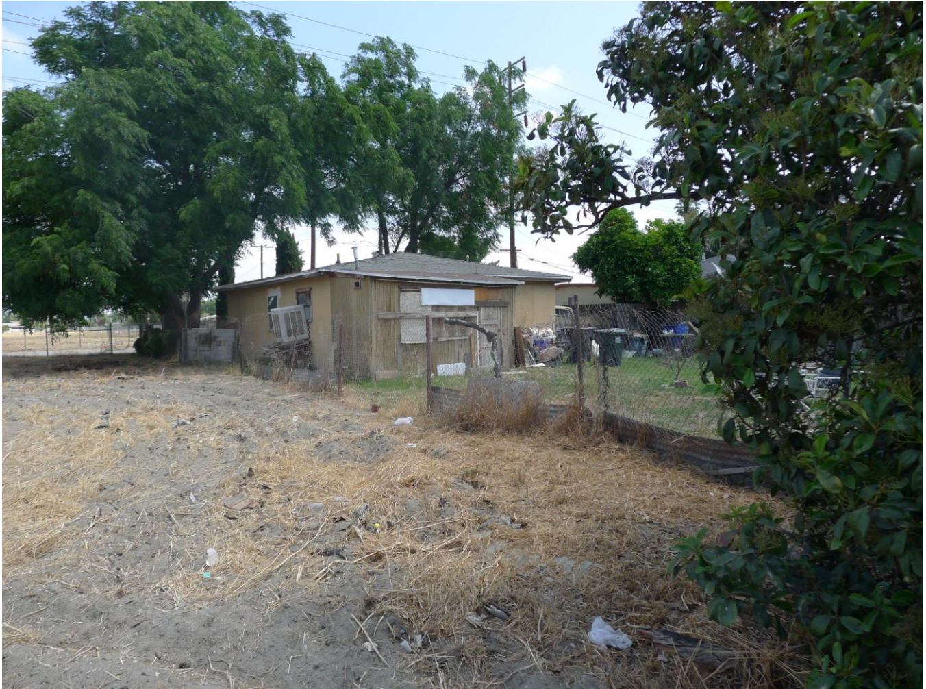
South elevation, facing northeast (photograph taken May 27, 2017)
