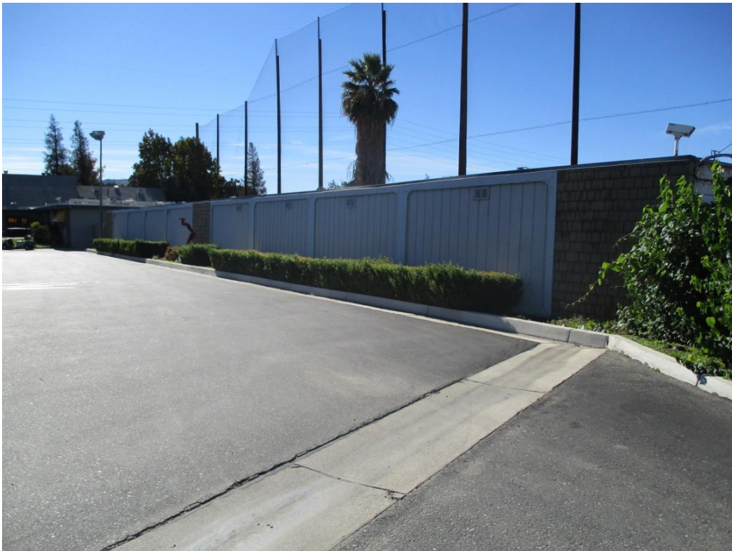
Figure 4-9 East side of golf cart storage building, facing southwest
