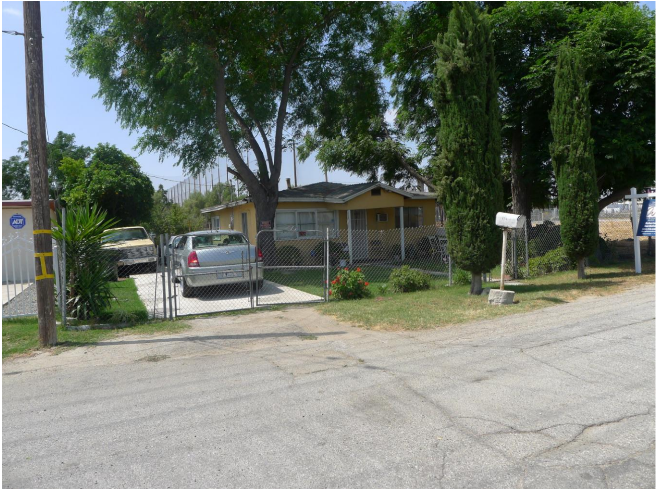
North elevation, facing south (photograph taken May 27, 2017)
