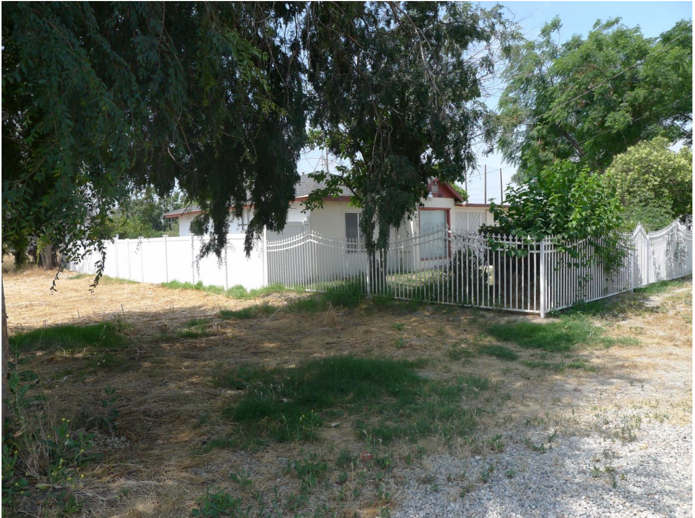
East elevation, facing southwest (photograph taken May 27, 2017)
