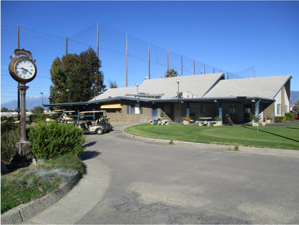
Figure 4-8 South side of clubhouse, facing northwest
