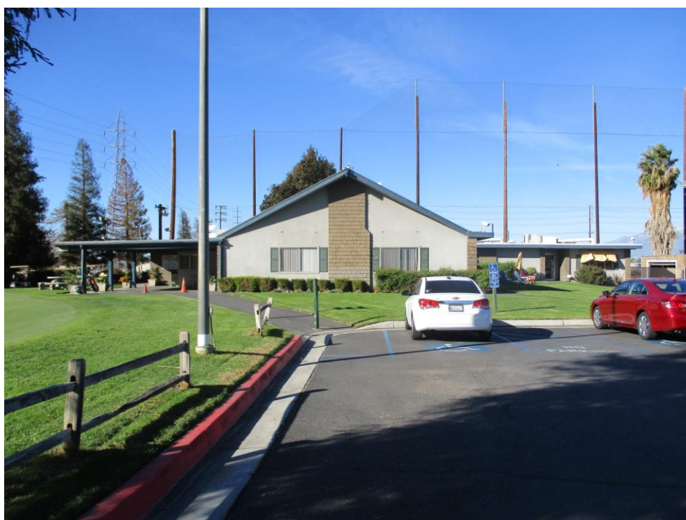
East elevation of clubhouse, facing west (photograph taken November 29, 2016)
