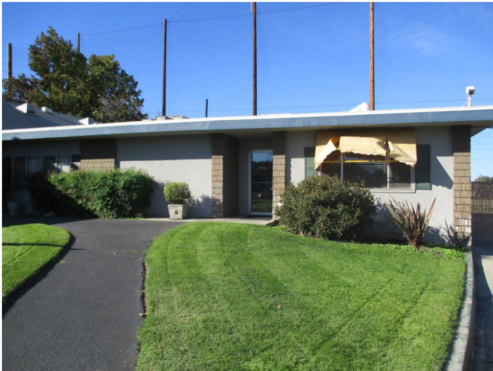
East elevation of clubhouse addition, facing west (photograph taken November 29, 2016)
