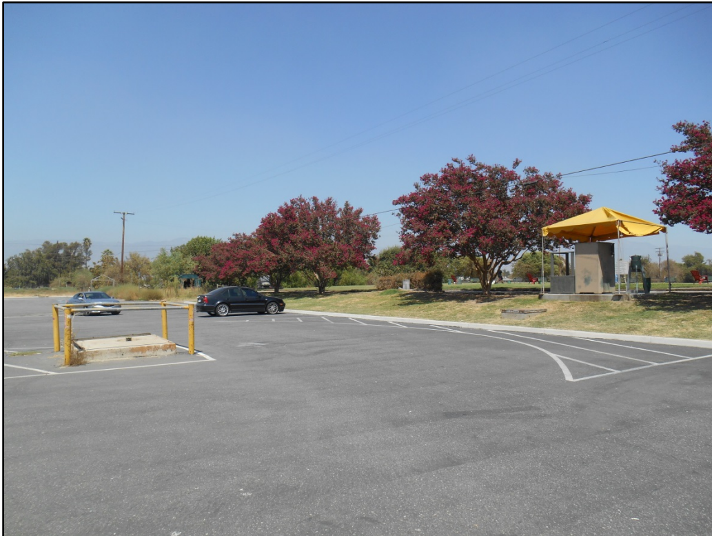
Photo 2 – Looking northeast at existing Thorne 9 well towards Dumas Street.
