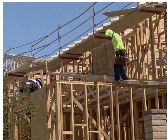
Construction workers building housing
