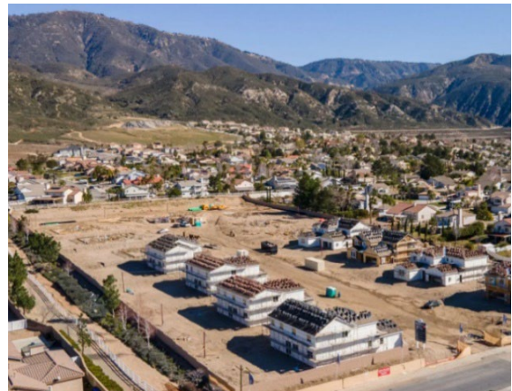
Belmont Collection Construction
