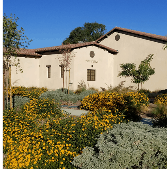
Casa Paseo, a 11,000-square-foot facility situated on approximately 3 acres in San Bernardino
